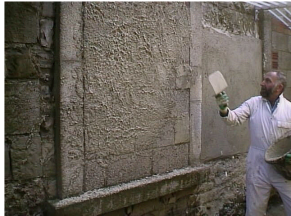
Above: Harling using the Harling Trowel
