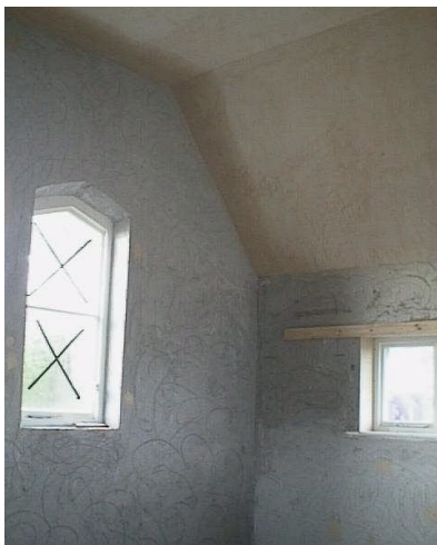
Above: Second coat of coarse stuff finished with a Devil Float
